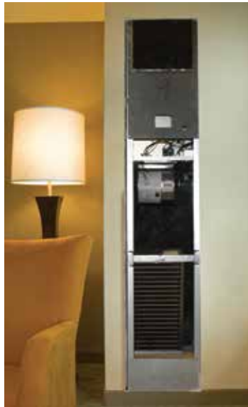
Remove surface components and trim drywall.
