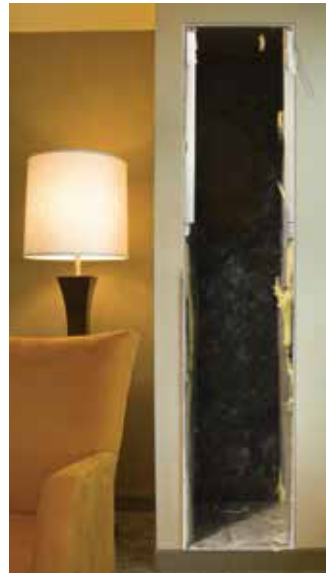
Remove internal components and trim cabinet edges.
